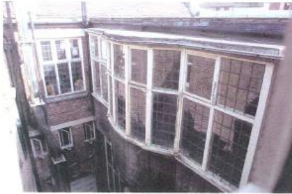
Repairing the fabric of the building
