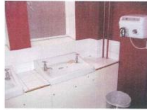
Renovating and increasing the number of toilets
