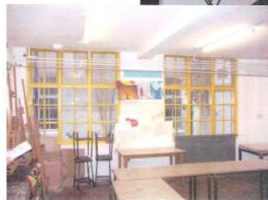
Refurbishing the art room and providing better lighting
